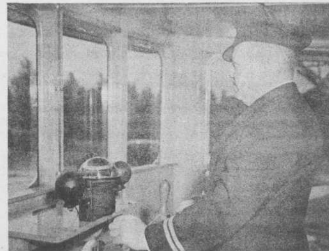
Captain Bradley at the wheel, sailed tug from contractor's plant to Port Weller.
