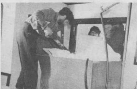
Each station presents a different problem in obtaining its water winter. At Isachsen, the men cut snow blocks which are carried to the sleds. The snow blocks are passed through a window into a room, snow is melted and the water is then pumped to an overhead tank; thus running water for showers and for the washing machine on wash day; I Ingram of Winnipeg, brings a snow block to the kitchen where cook Jim New York says "Just one today". Other stations get water from the blocks of glacier ice.
