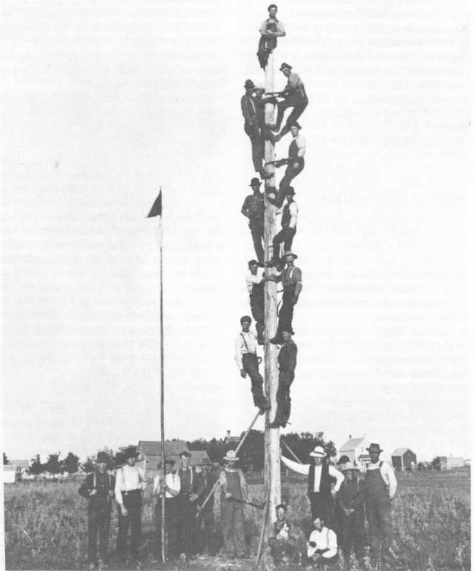
Putting up Government telephone lines through the rural district. (Photo: Department of Energy, Mines & Resources - National Archives of Canada)
